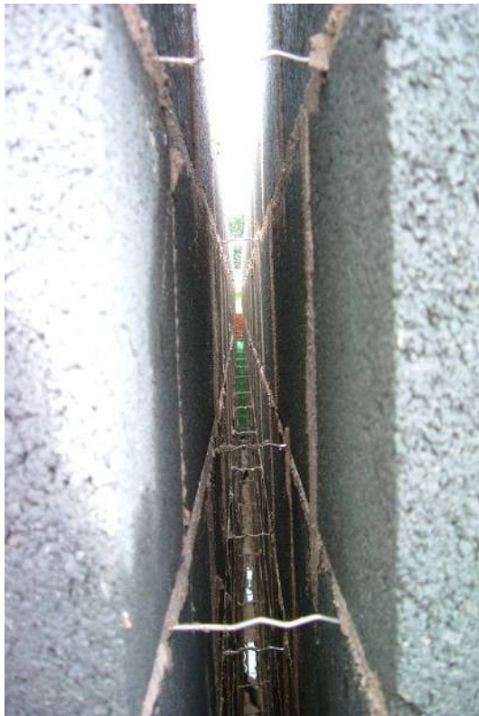
Stamford Brook – thermal envelope defects – convective bypasses (Lowe et al 2007)
